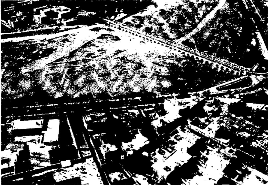
6.8 Si-o-Seh Pol, or the bridge of thirty-three arches, on the Zayandeh river, is one of the most famous of Isfahan's bridges. It was commissioned in 1602 by Shāh 'Abbās I. The bridge is 295 m long and 13.75 m wide
